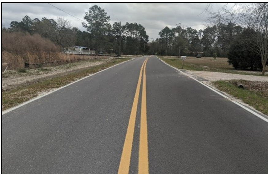
Street, Flood, and Drainage Improvements
